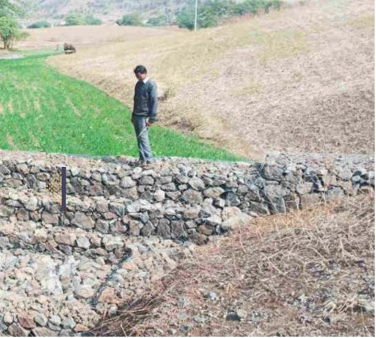
Gabion structure has restored the soil by checking the silt, increase soil moisture and enabled wheat crop production in the restored gulley in Thetham village under NABARD Watershed Development Fund Project in Jhabua, Madhya Pradesh
