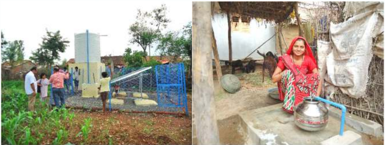
Figure 2. The solar drinking water system installed in 21 hamlets in Dahod district of Gujarat.
