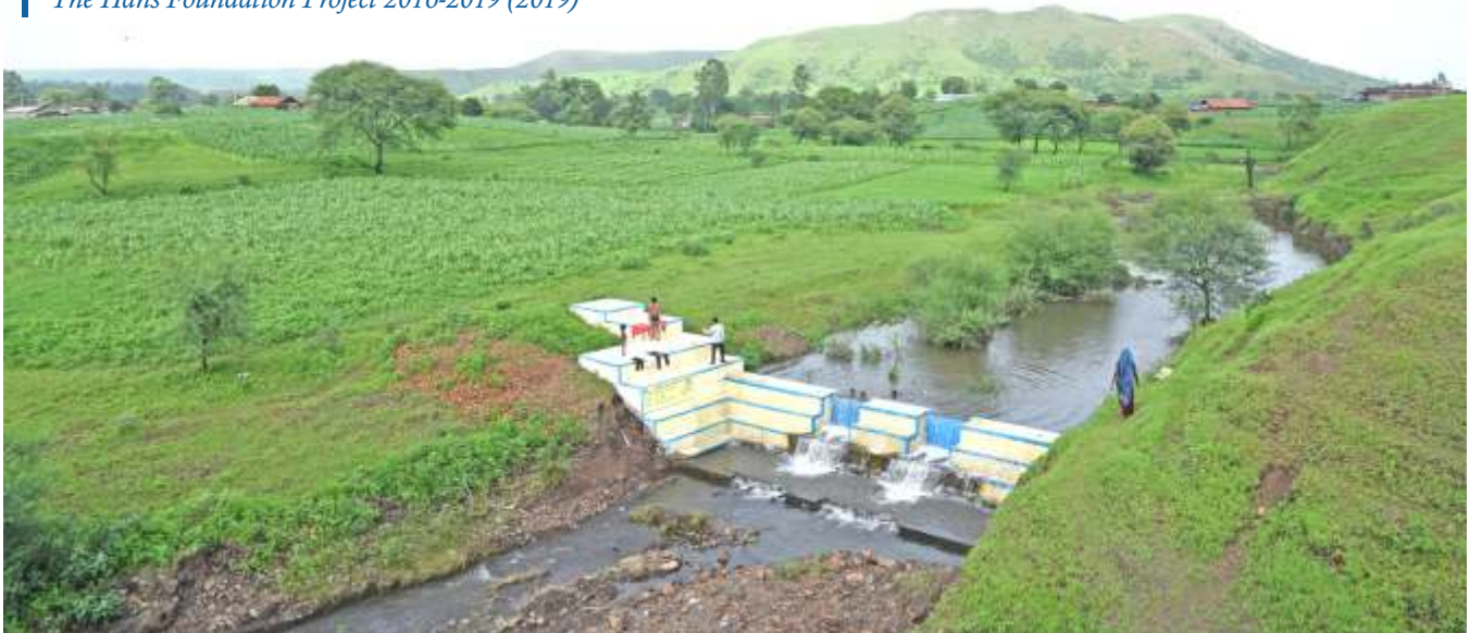
Check dam constructed at Thetam village of Jhabua, Madhya Pradesh under The Hans Foundation Project 2016-2019 (2019)
