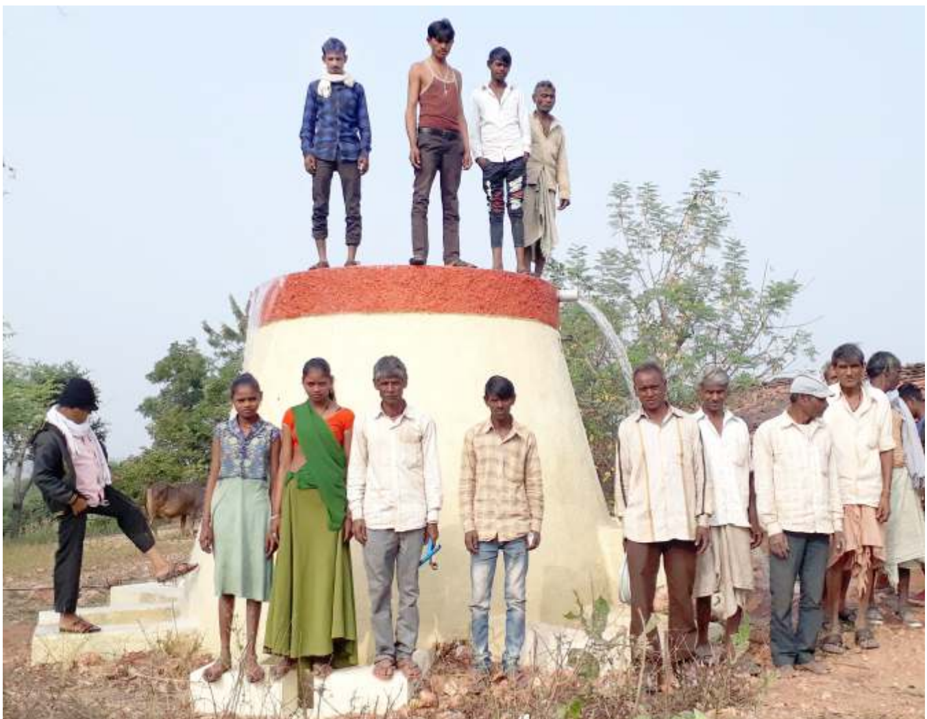
Happy farmers of Jogiwada Lift irrigation scheme, Gangad Talai block of Banswara, under RKVY, Rajasthan
