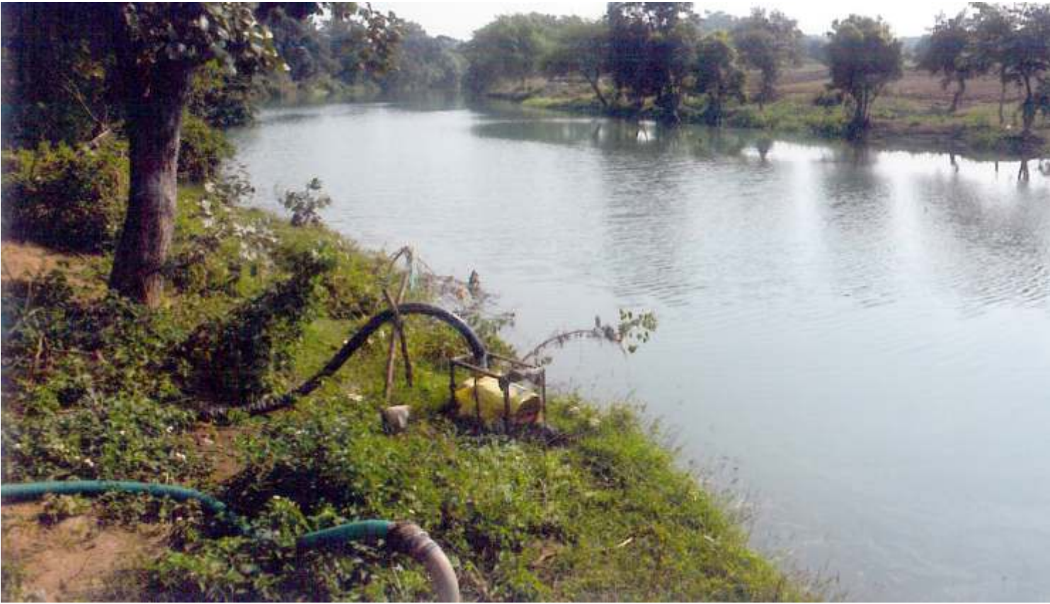
Chaurikhurd -1 check dam across river Chacharni, Tehsil Gangdhar, District Jhalawar with the support of Agriculture Department Rajasthan (RKVY-Project)
