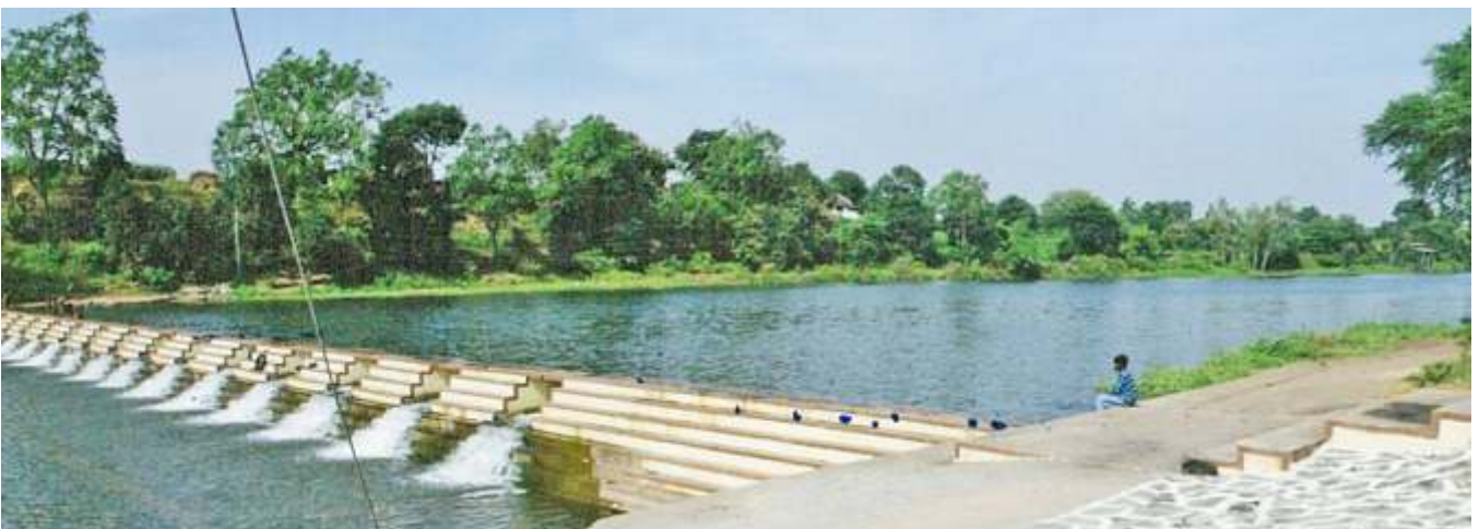
Bhimkunda-1 check dam across river Patri, Tehsil Thandla, District Jhabua with the support of Coca-Cola India Foundation, New Delhi.
