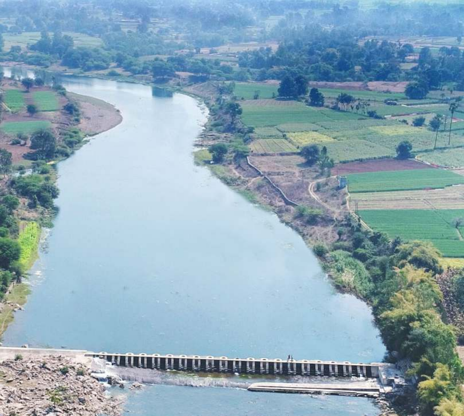
Dhabudi Check dam across river Hadaf, constructed in the year 1996 with the support of DRDA (JRY-III) in Limkheda Taluka of Dahod District, renovated in the 2019-20 under Aspirational District Dahod with the support of ONGC CSR Fund
