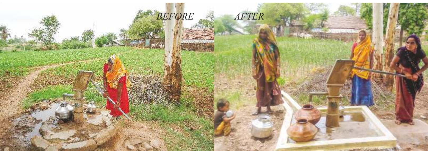
Hand pump reparations (supported by Axis Bank Foundation) at Village, Jambua (Kalitalai Faliya), Taluka Garbada, Dahod
