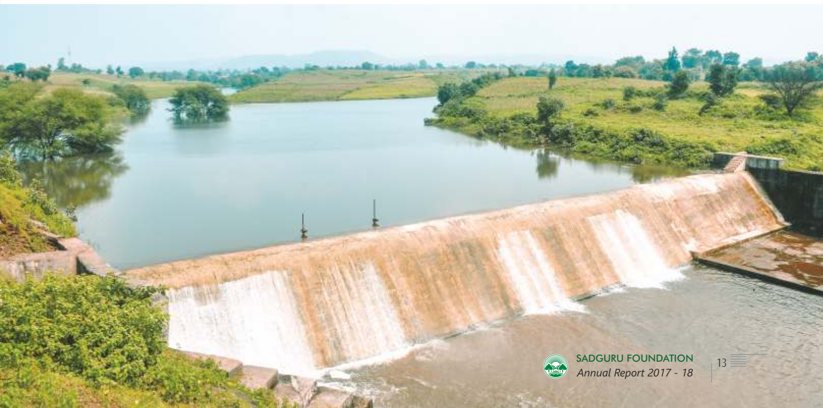
Vajwa Amba check dam with storage capacity of 17 mcft, across river Hiren in district Banswara under RKVY project Rajasthan, co-funded by AXIS Bank Foundation, Mumbai
