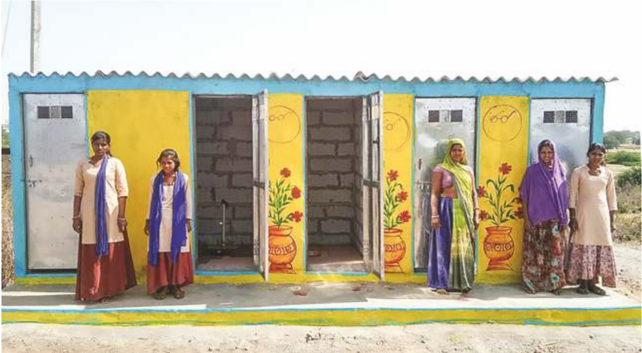
Sanitation block constructed at village Balasindur, Banswara, Rajasthan, under the model village of Axis Bank Foundation. 78 sanitation block constructed recently in this village
