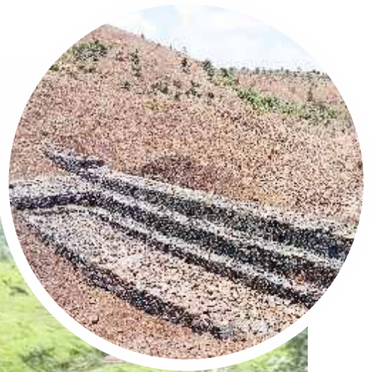
Gabion constructed at Dhamanjar Village under EY foundation Harit Dhara project supporting stabilization of drainage system and increase recharge of rainwater and vegetation in upstream and downstream
