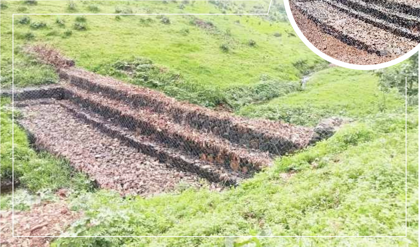
Gabion constructed at Dhamanjar Village under EY foundation Harit Dhara project supporting stabilization of drainage system and increase recharge of rainwater and vegetation in upstream and downstream
