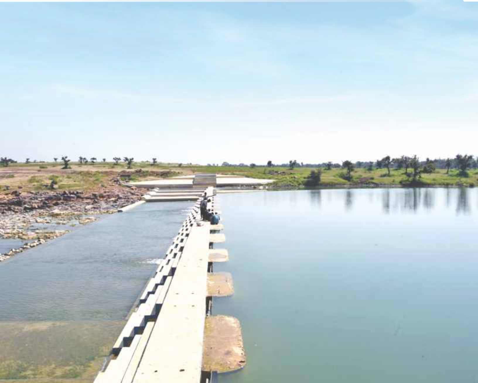
Karnakhedi Check dam implemented across river Kilol in Tehsil Gangdar, under RKVY-Jhalawar Project with storage capacity of 5 mcft, Potential created for irrigation is 175 acres of 60 house hold.
