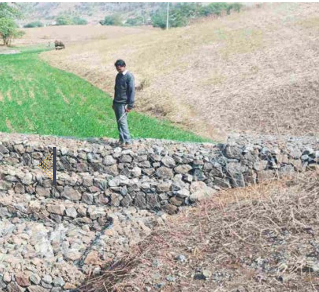
*Gabion structure has restored the soil by checking the silt, increase soil moisture and enabled wheat crop production in the restored gully in Thetham village under NABARD Watershed Development Fund Project in Jhabua, Madhya Pradesh*
