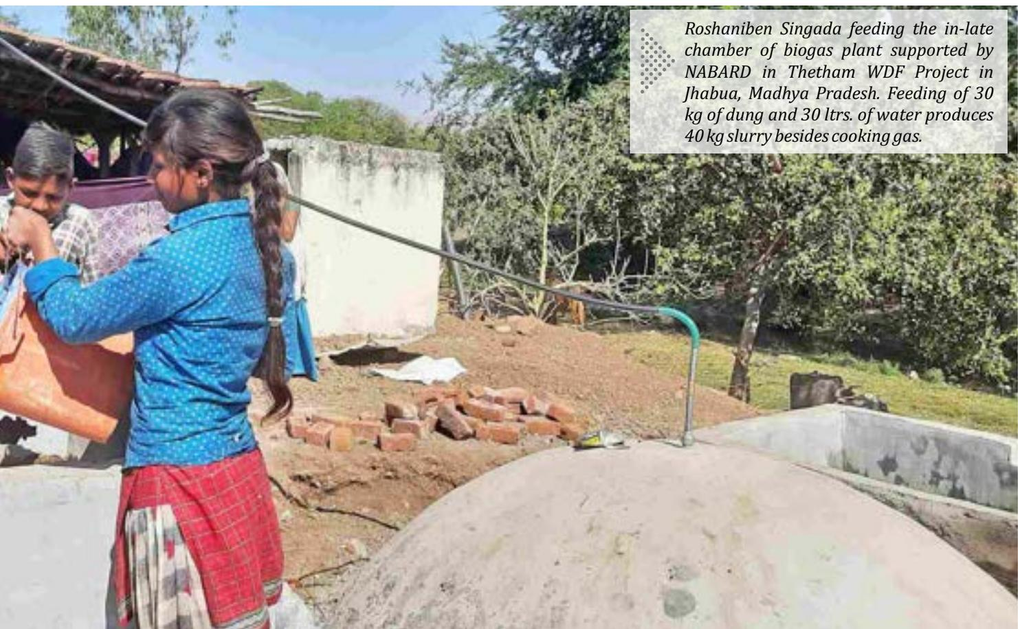
*Roshaniben Singada feeding the in-late chamber of biogas plant supported by NABARD in Thetham WDF Project in Jhabua, Madhya Pradesh. Feeding of 30 kg of dung and 30 ltrs. of water produces 40 kg slurry besides cooking gas.*
