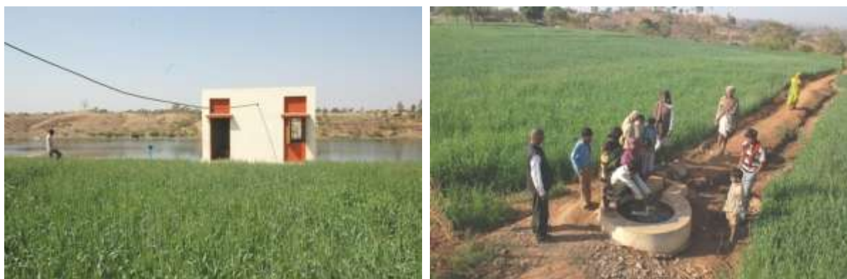
Community managed lift irrigation scheme at village Muniya Khunta and Jalampura, Banswara, Rajasthan constructed under the present RKVY project.
